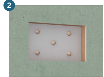
2 Fix Gib/Villa Board, dry fit niche, remove and apply adhesive
